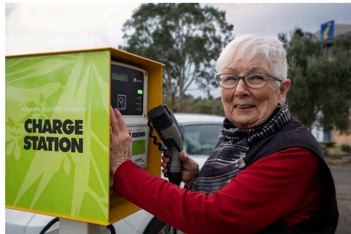
Electric vehicle charging infrastructure at the McLaren Vale Visitor Centre
