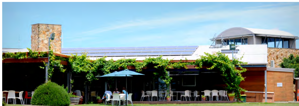
The McLaren Vale Visitor Information Centre Green Hub
